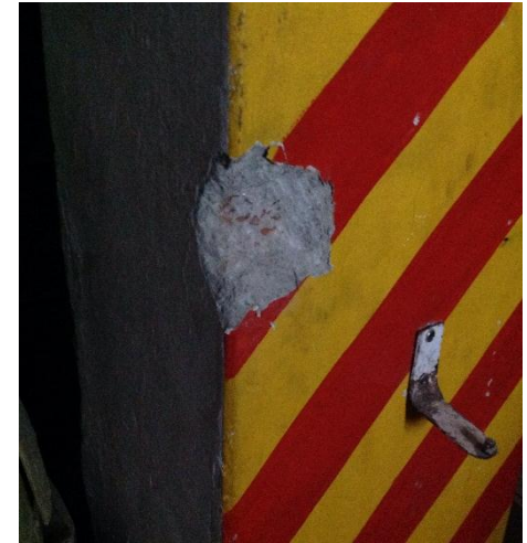
Checked Ground Floor Column – Brick Chips
