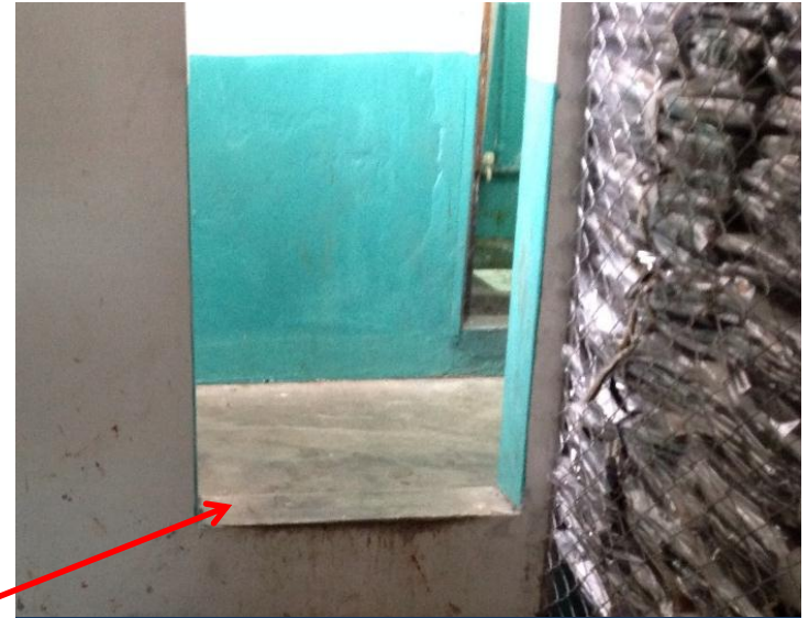
Toilet Floor Build up
