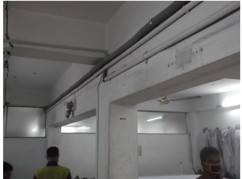
R.C. Beams and solid slabs typical at each floor – with deeper beams at u/side of 2 nd floor
