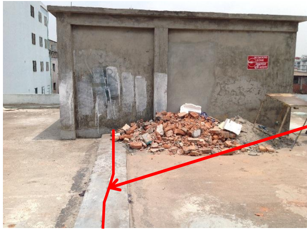
Building Movement Joint
