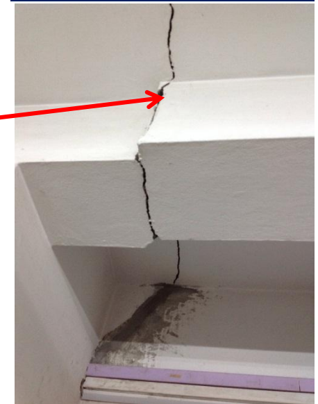
Movement joint evident at all floors
