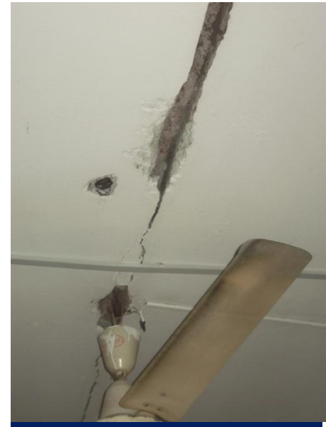
Movement joint evident at all floors
